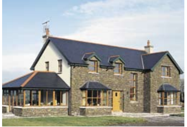
This house features Munster Joinery High Performance Light Golden Oak windows in Casement and Tilt & Turn. Matched with Munster Joinery multi-point locking door set. Also featured is a light oak sun room with Munster Joinery Casement Windows.
