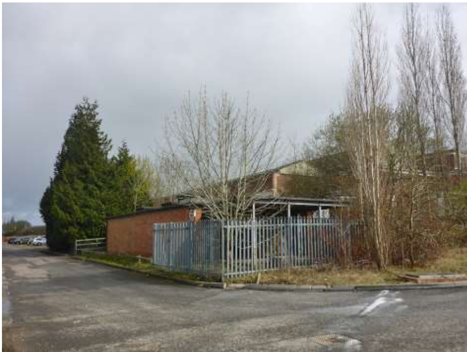
The Old Armoury looking east from Artisan Road.
