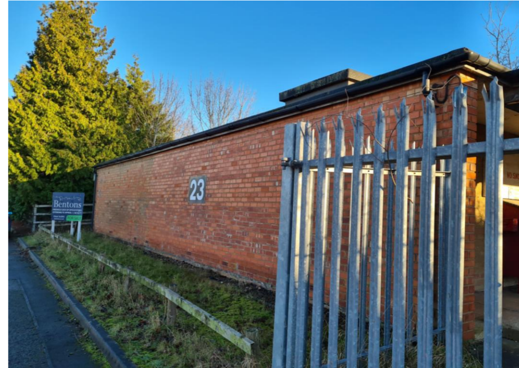
Unit 23 to be demolished
