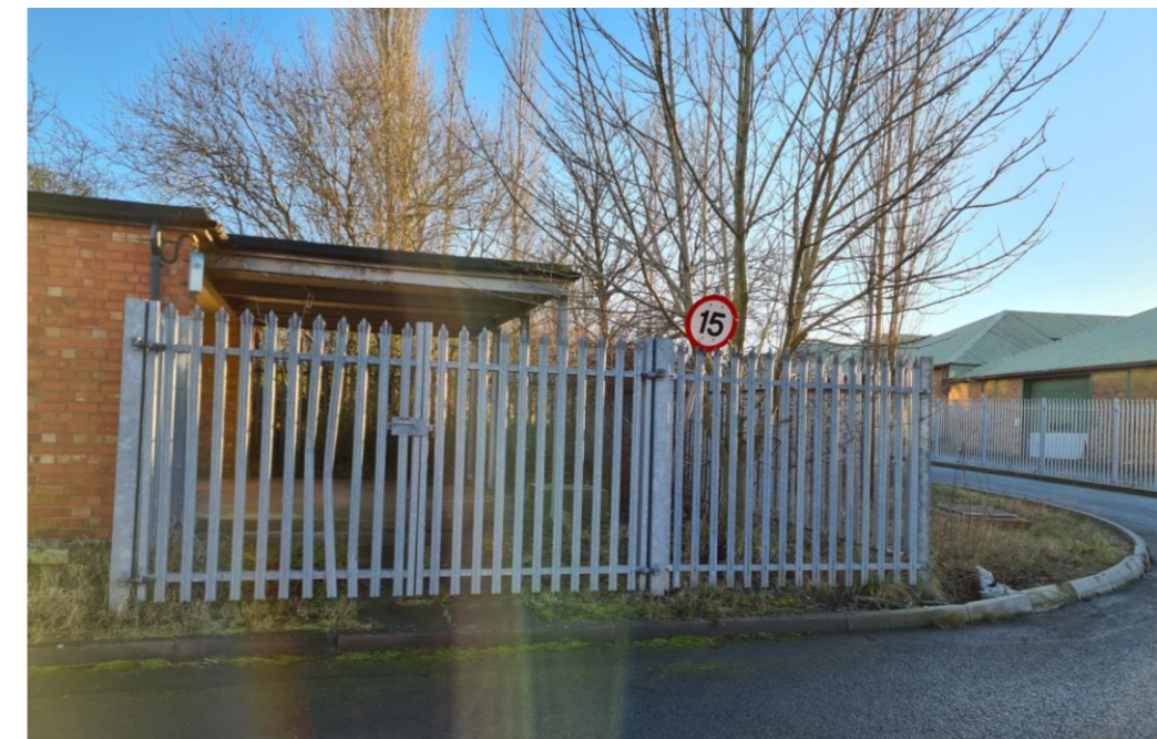
View western end of site – secure compound
