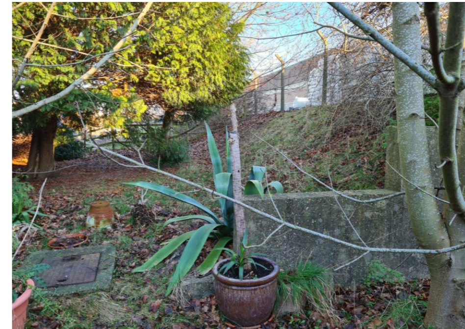
Bank and retaining wall to southern boundary
