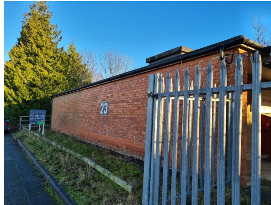
View of unit 23 to be demolished.
