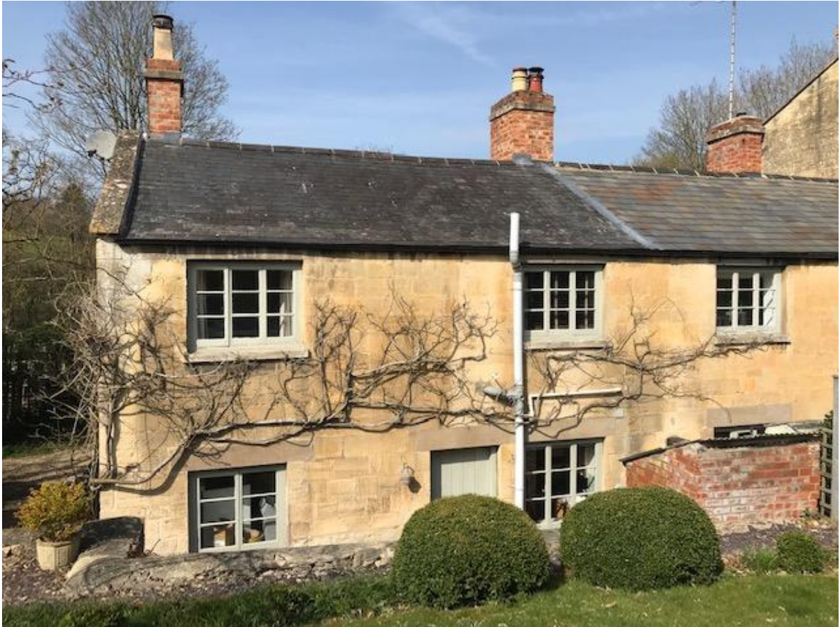
4 Coates Mill Cottages. Rear Elevation
