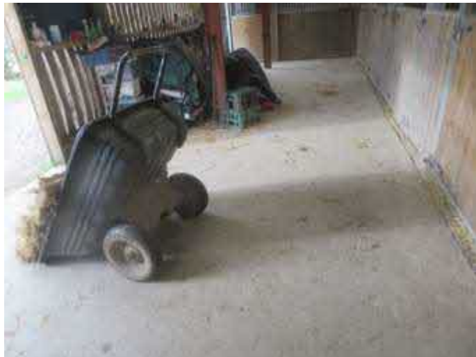
Solid floor in steel barn
