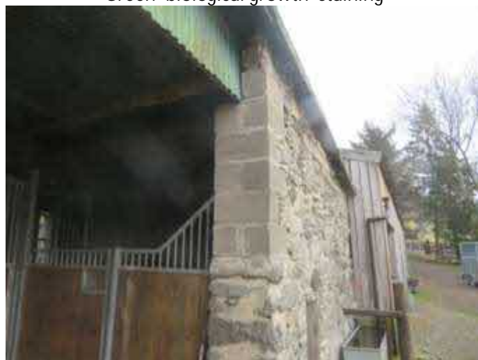
Sections rebuilt in concrete block
