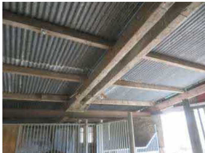
Joists and central crossbeams to stone barn
