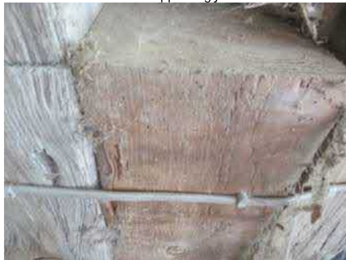
Active beetle attack to crossbeam
