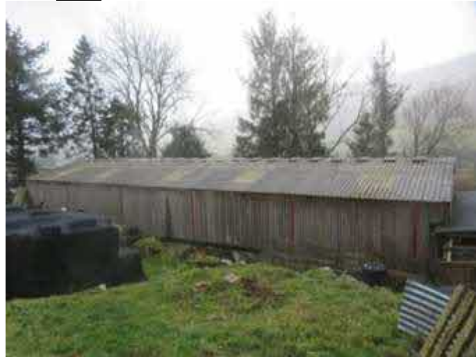
Assumed asbestos cement over steel framed structure
