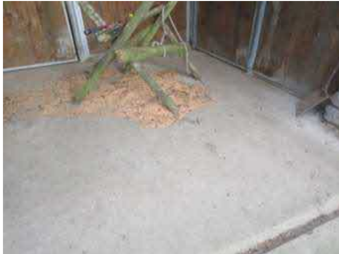
Solid floor in stone barn
