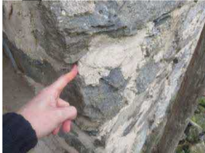
Re-pointing with cement mortar
