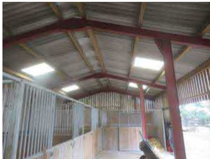
Steel trusses supporting structure
