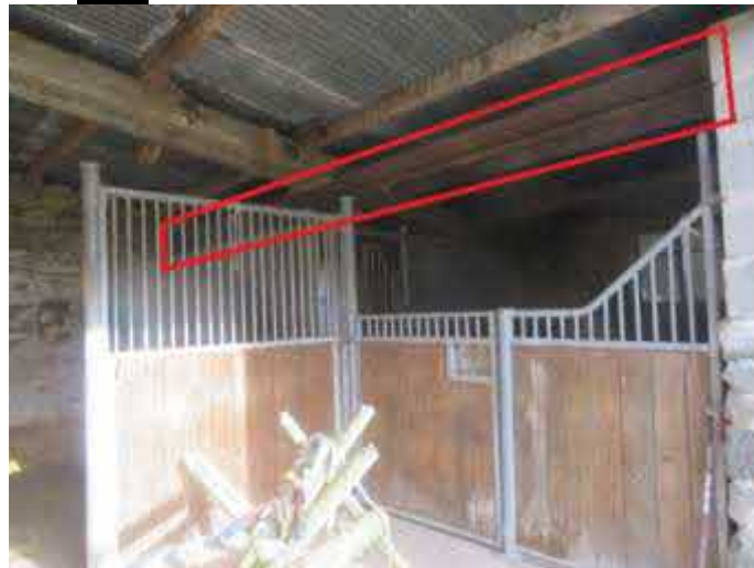
Steel supporting joist
