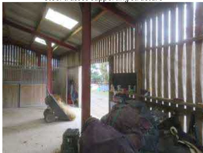
Timber panels between trusses
