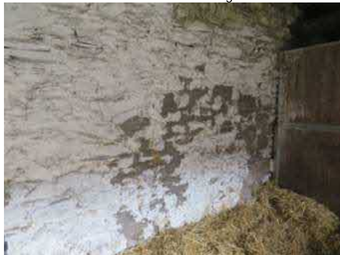
Lime washing to inner wall
