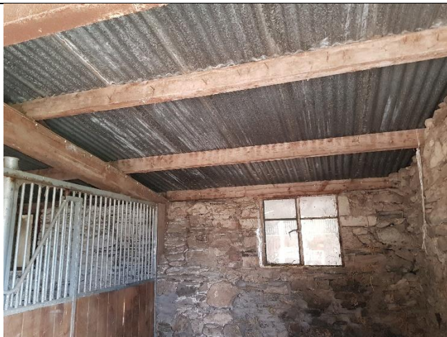
Roof structure within.
