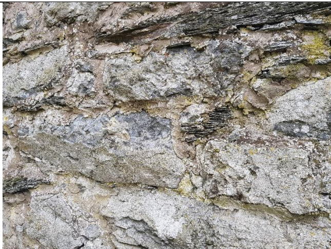
External stonework is mostly well-sealed with cement.
