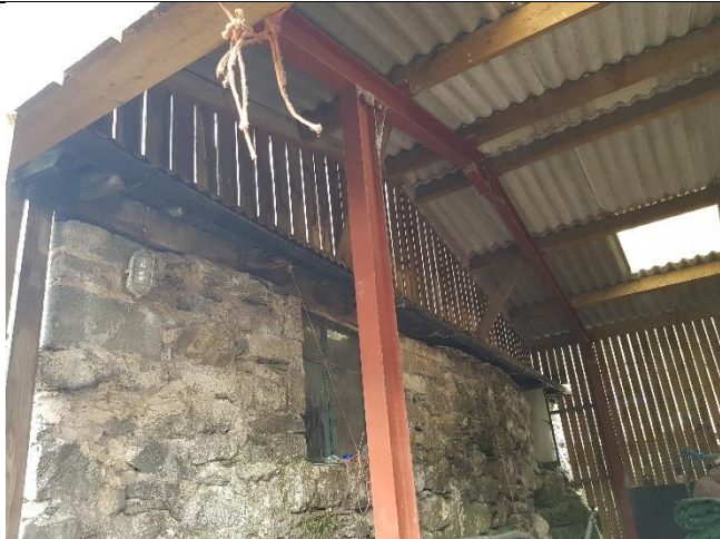
Junction between stone barn and adjacent steel framed stable block.
