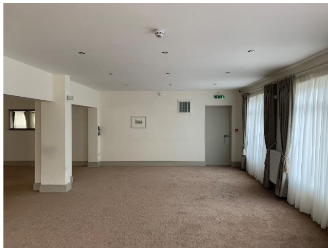
Existing Internals – Function Room
