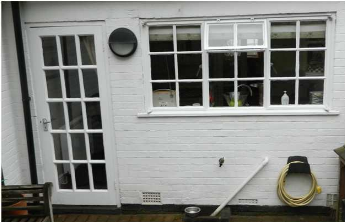
Existing rear kitchen window and door to be replaced
