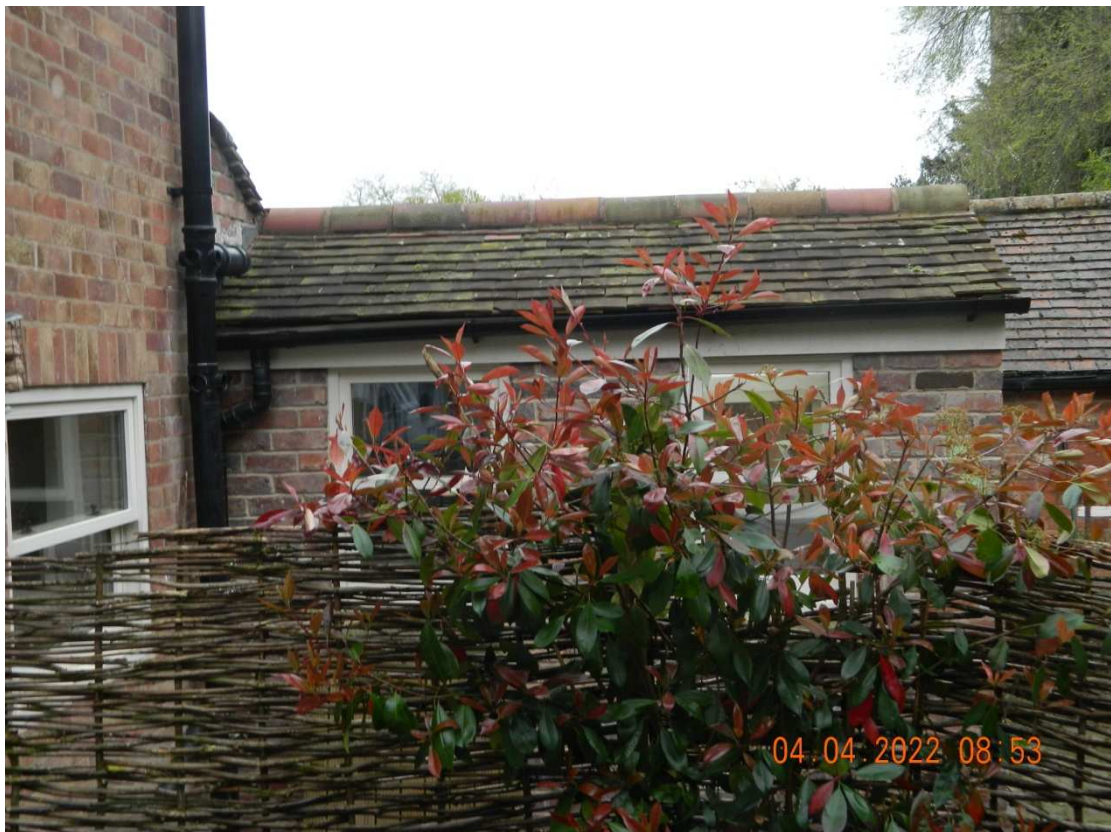
Photograph of No24's kitchen window and walkway extension dating from 2018
