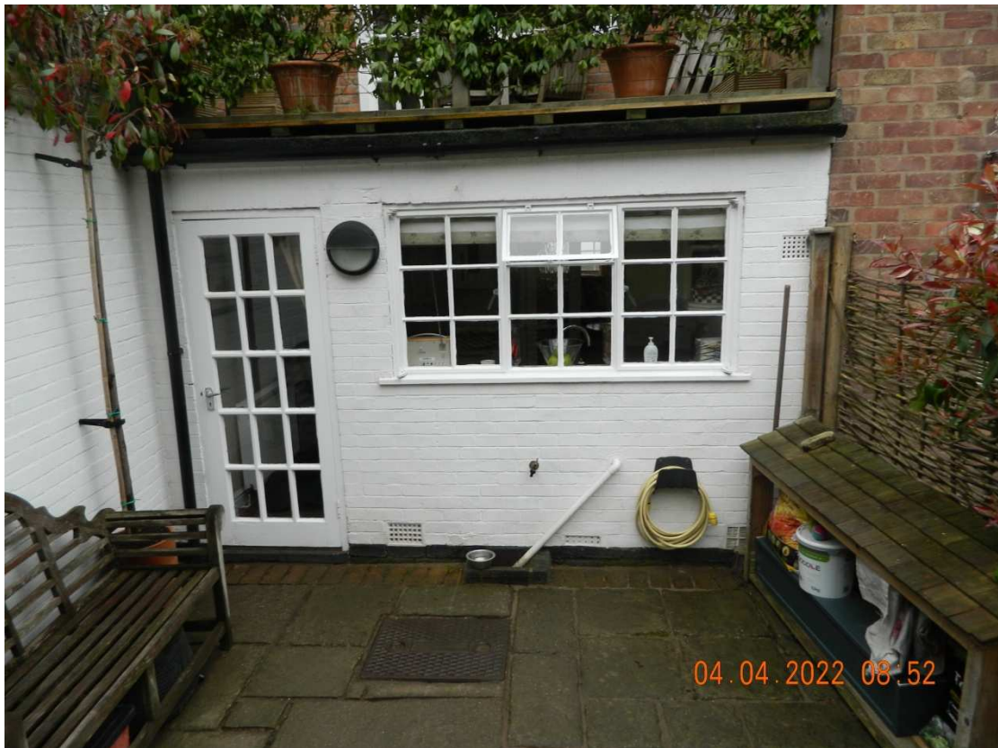
Photograph of existing rear elevation
