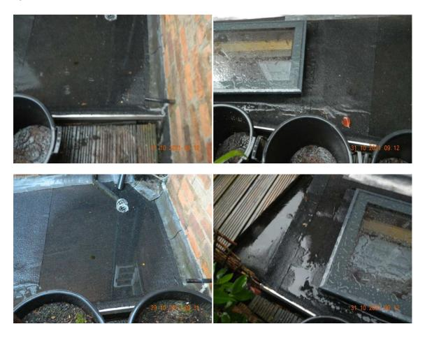
The proposed new 225mm tall upstand will be installed in the same location, but extended by 80mm in length towards 20 Mill Street's step up to the property's back-ward sloping balcony. The height of the new upstand will be uniform, except at this 200mm step, where it will be 25mm tall.
