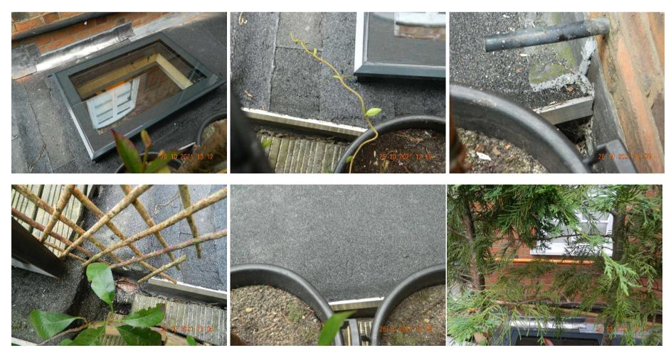
The slope of new roof fails to gather and transport rain/surface water to the other end of the flat roof and dispose of it via the installed roof drain gully inlet. Instead, water is allowed to pool on various areas of the roof, including next to the 22 Mill Street upstand/boundary marker.
