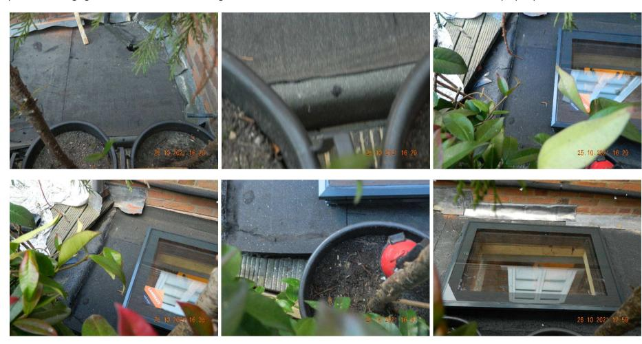
Boundary infringement. Aluminium finishing trim attached to top of 22 Mill Street upstand to cover where new felt had been lapped over it.
