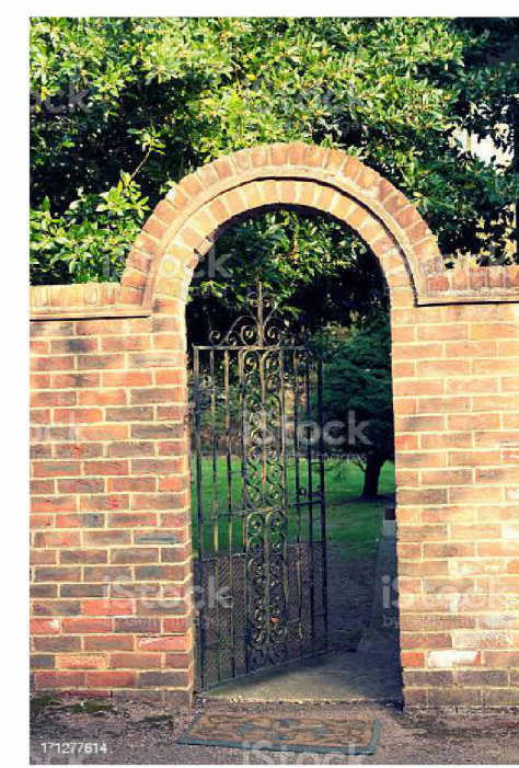
Example of arched brick opening
