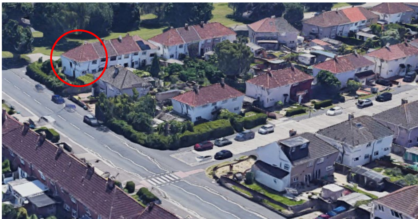
Hip-to-gable and rear dormer extension at 247 Ullswater Road (application site circled)
