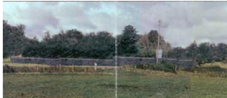
A view from south of the site towards the original quarry buildings and access after the restoration
