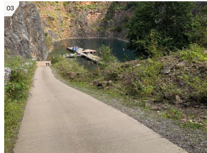
View of the lower section of the existing quarry haul road
