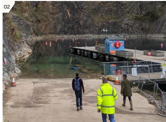
02 View of the existing slipway from the south
