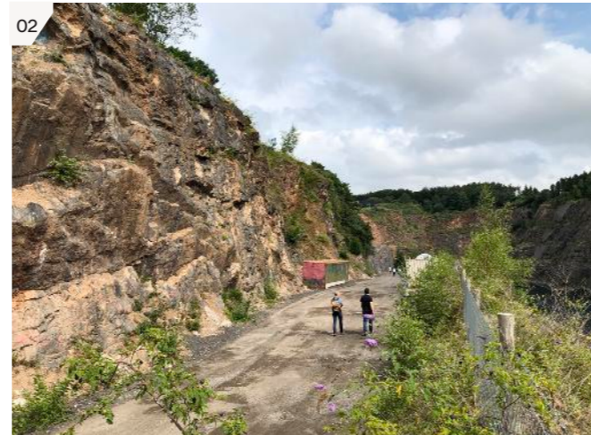
View of the top section of the existing quarry haul road
