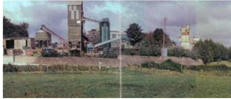
A view from south of the site towards the quarry plant area and access prior to restoration
