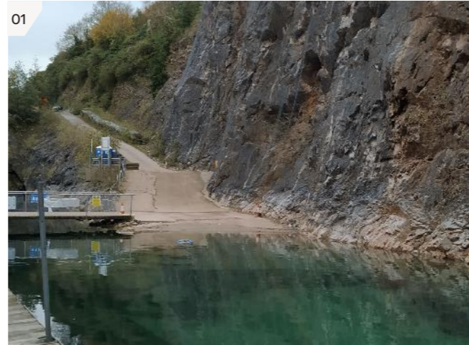
01 View of the existing slipway from the north
