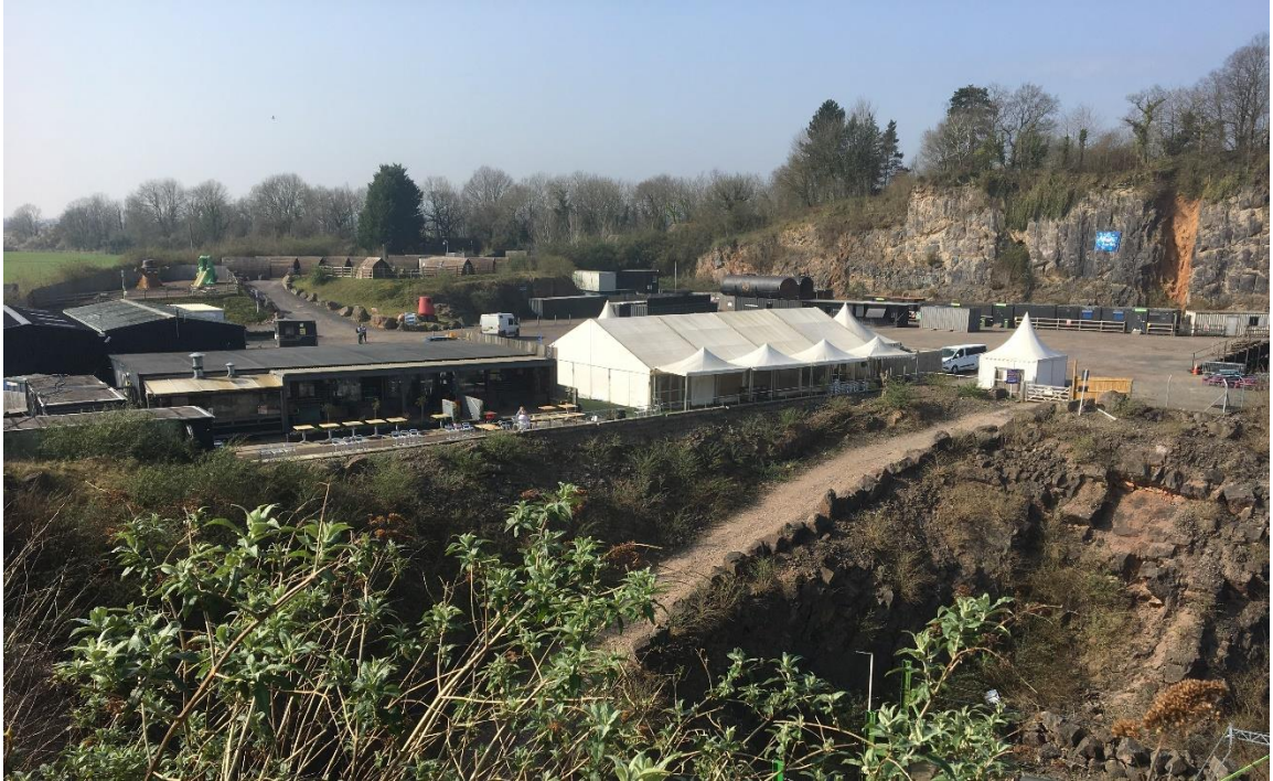
Existing site entrance, buildings and car park
