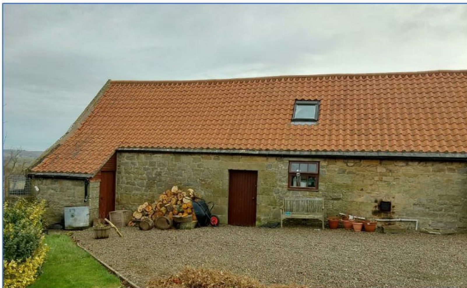
North Elevation – stables area
