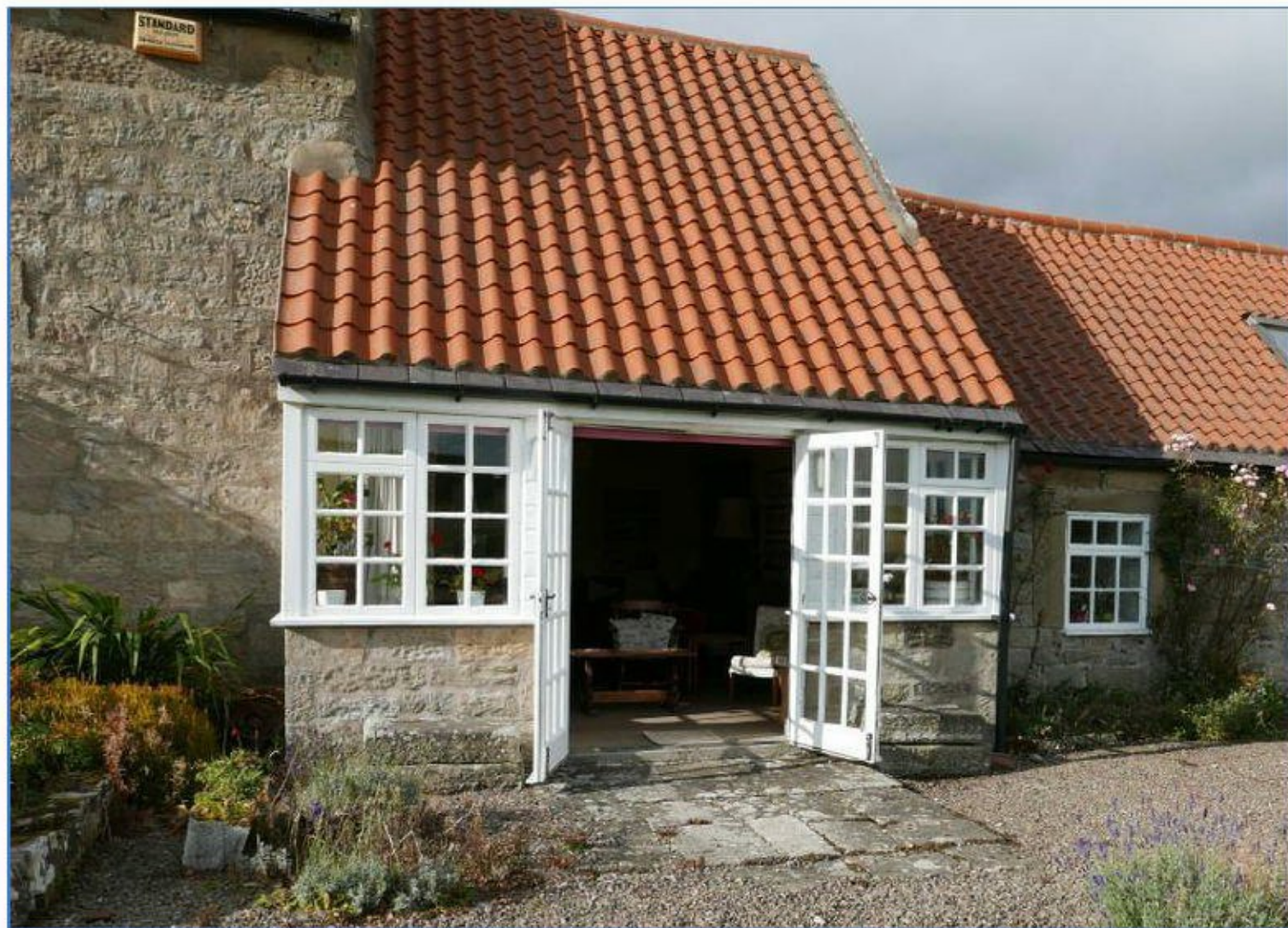
Doors to replace in cart shed area
