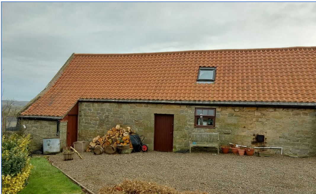
North Elevation – stables area
