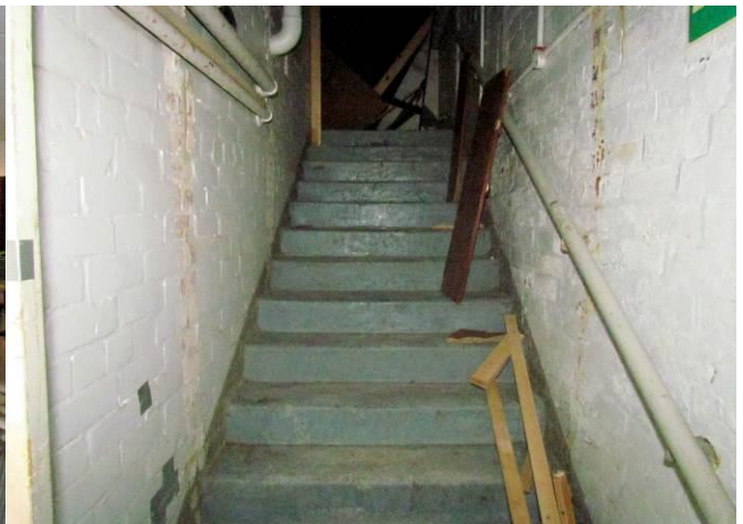
Staircase to Basement
