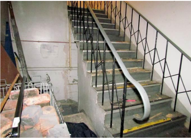
Staircase in North Corner
