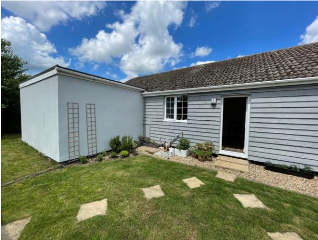
Rear South East Elevation
