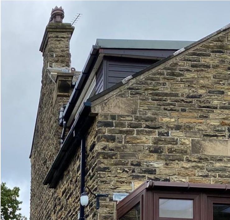
Dormer side view
