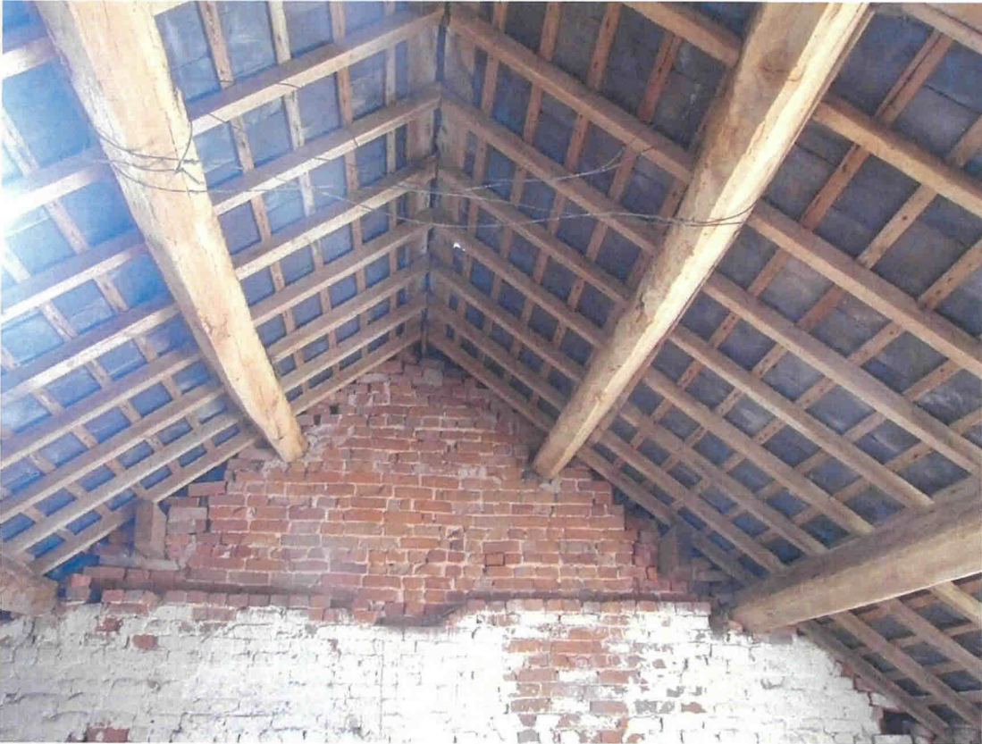
Barn A roof structure right gabel.
