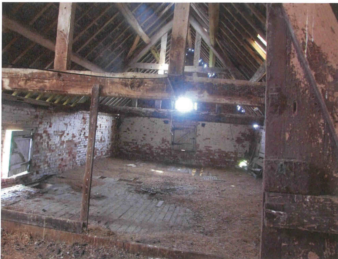
Barn B internal first floor.
