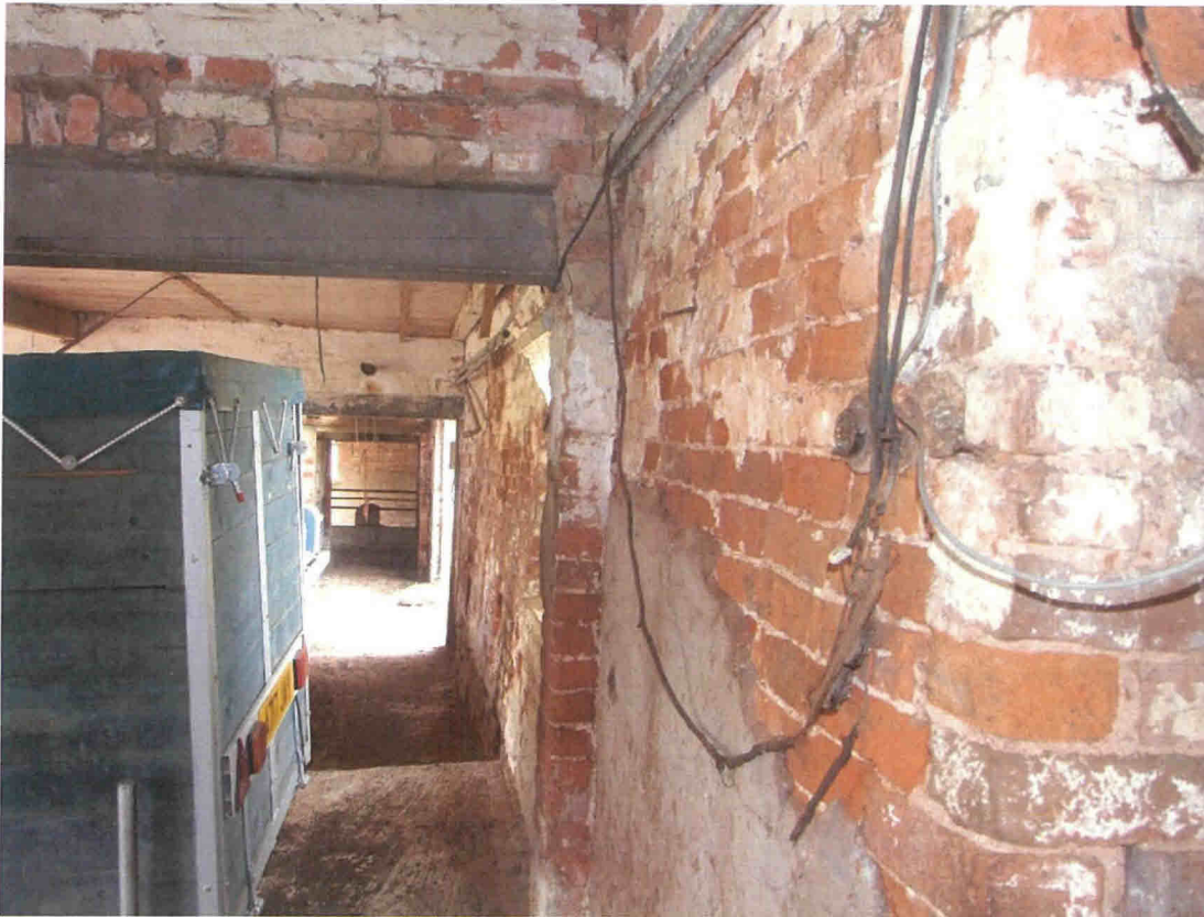
Barn A rear wall internal
