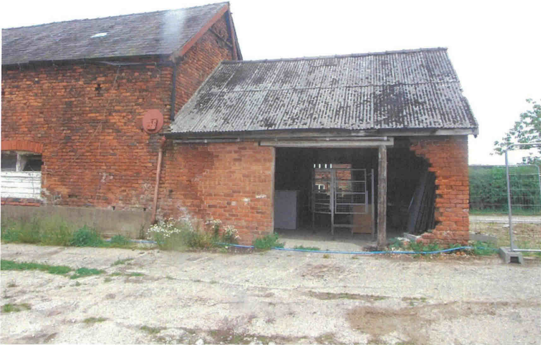
Barn A Rear elevation single element.
