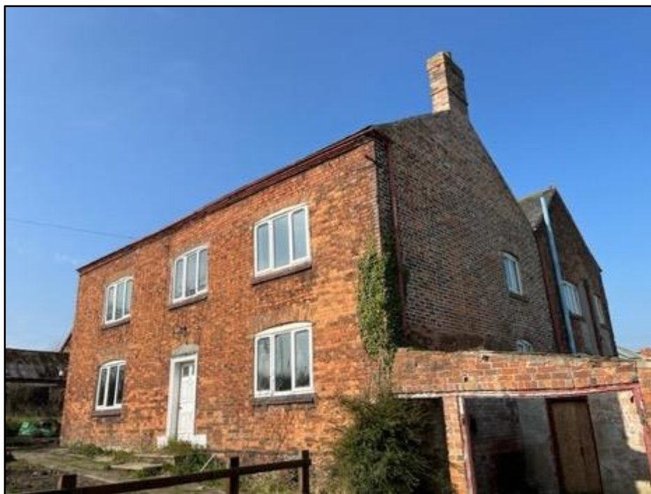
Fig 3: The northern gable of the building is in good condition.
