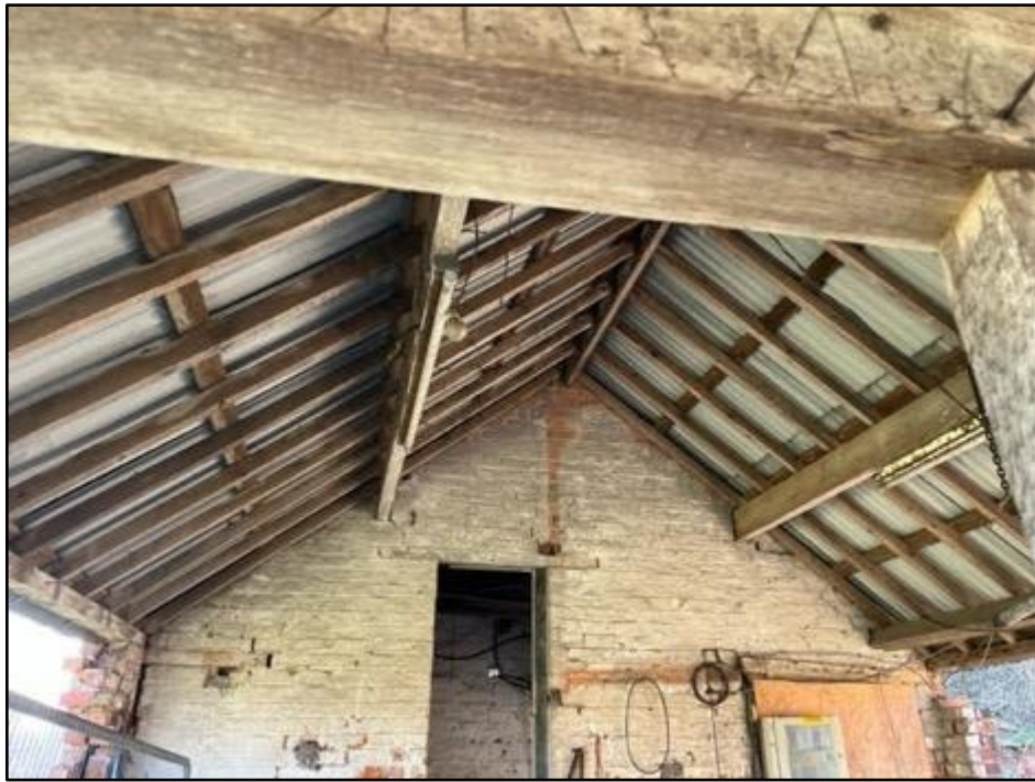
Fig 6: An internal view of the outbuilding.
