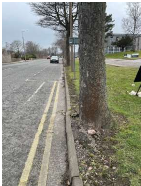
Photo 32 - View of T58 proximity to kerb
