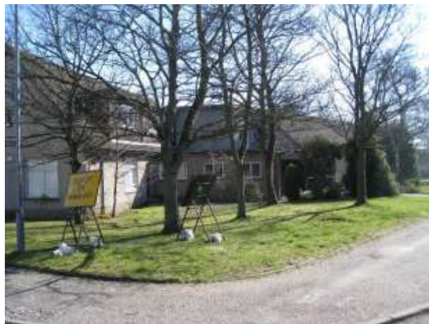
Photo 4: Sycamore trees within the grassland to the northwest of the building.
