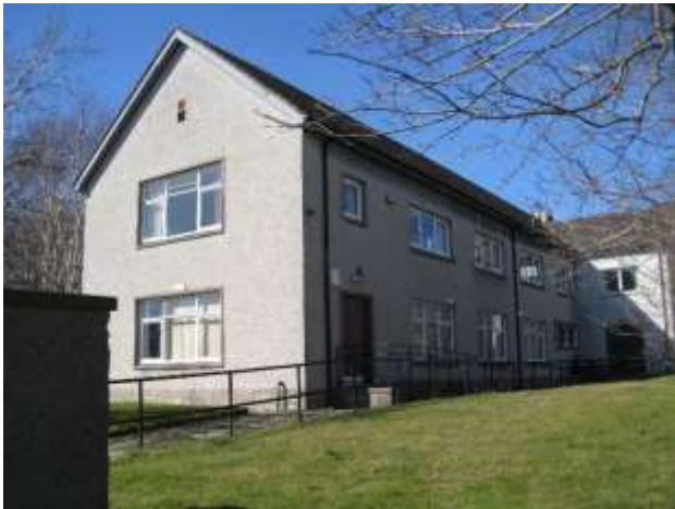
Photo 9: Two-storey section of the building at the eastern end
