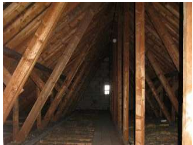
Photo 12: Typical internal structure of the building.
