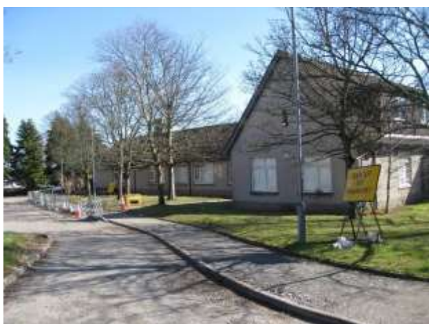
Photo 5: Cherry and sycamore trees to the north of the building.
