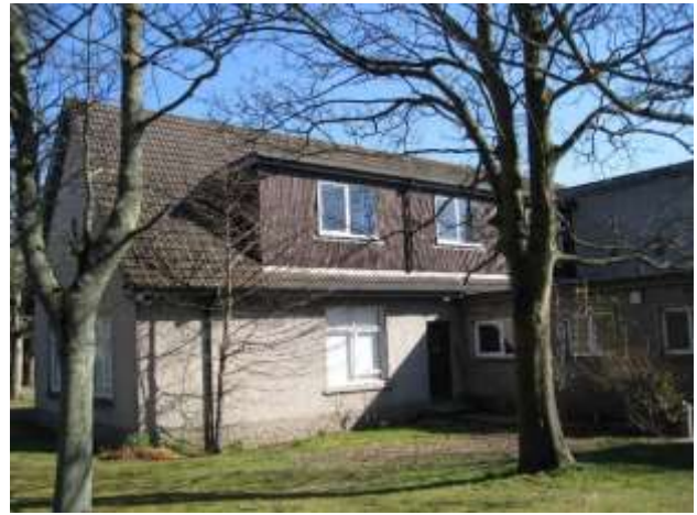
Photo 10: Northern wing of the building has rooms in the roof space and dormer windows.
