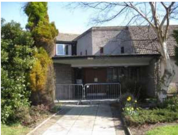
Photo 11: Flat roof section at the main entrance to the building.
