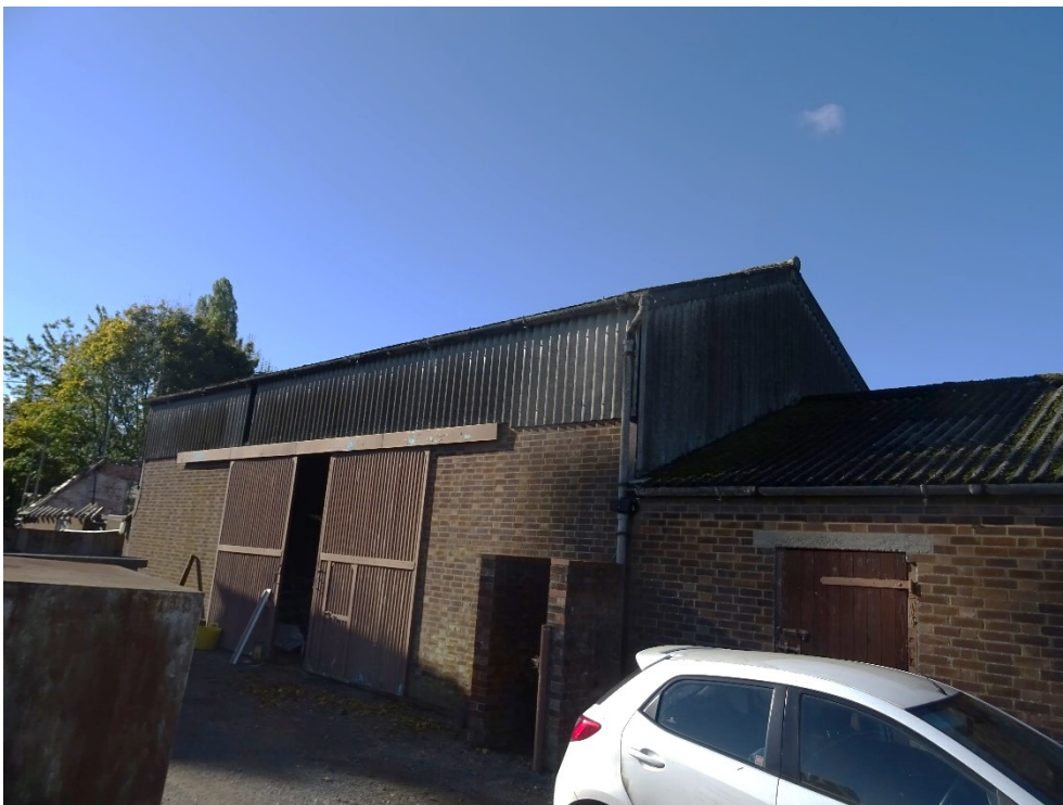
Photograph 6; Building 2 north-east aspect
