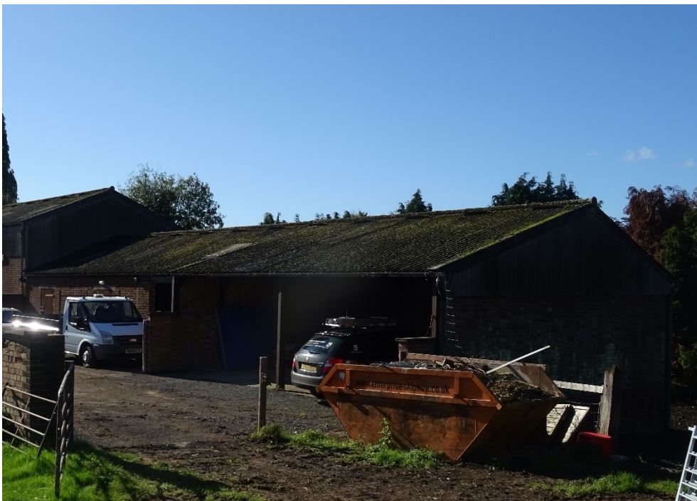
Photograph 4: Building 1 north east aspect
