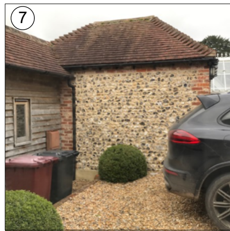
Natural flintwork laid in natural mortar
