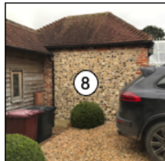
8 Natural flintwork laid in natural mortar
