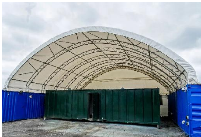
Proprietary covers between storage containers
