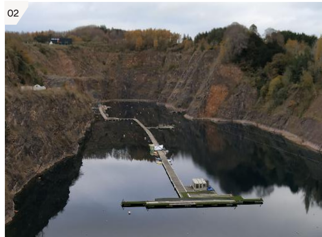
02 View of the existing pontoons from the southern quarry wall
