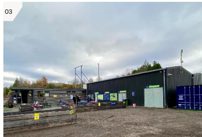
Retained and renovated black metal sheds with pitched roofs
