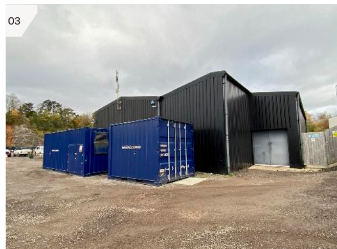
View of the storage building and hyperbaric chamber containers.
