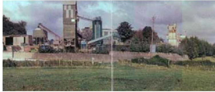
A view from south of the site towards the quarry plant area and access prior to restoration
