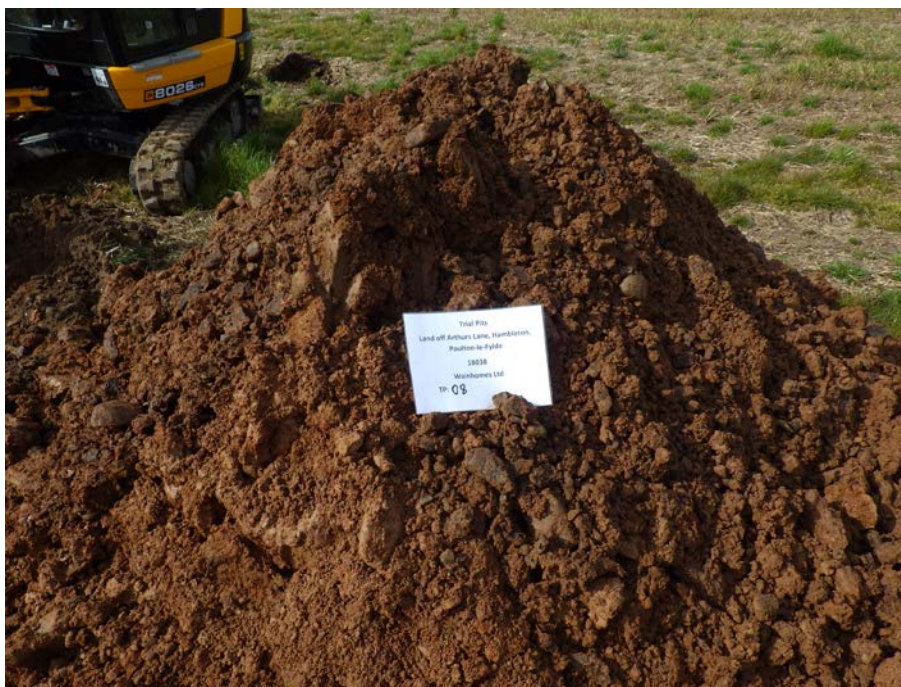
Photo 16 – Arising's from Trial Pit 08
