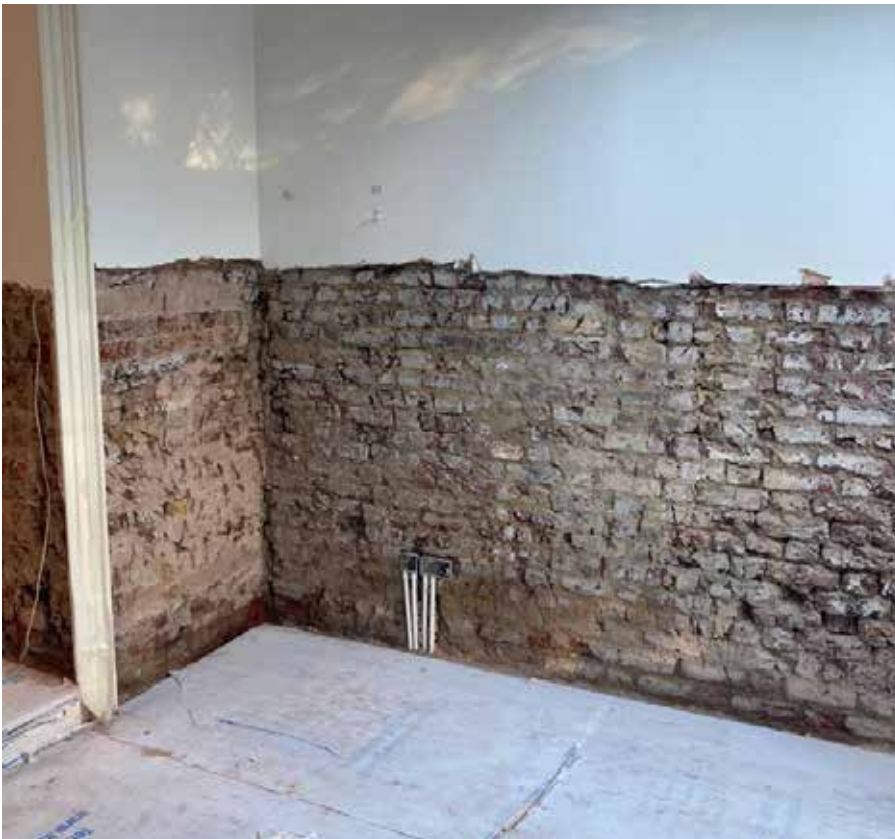
above , raised planter to front forecourt in poor condition and requiring repair. left , lower ground floor has signs of damp and require more invasive refurbishment works.
