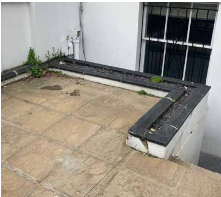
inside wall and coping removed only
