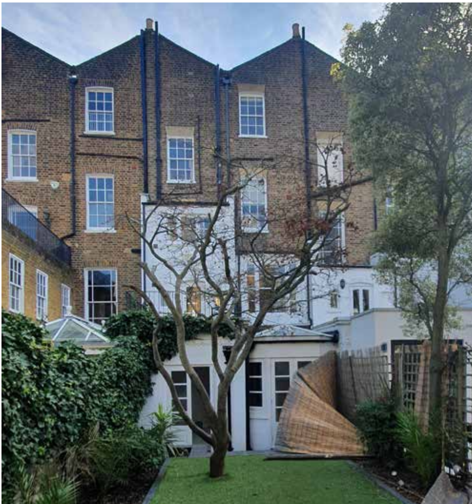
Rear elevation showing rear conservatory added in 1998
