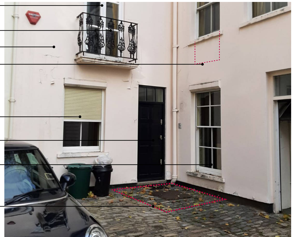
Rear View From Eaton Mews North Looking South
