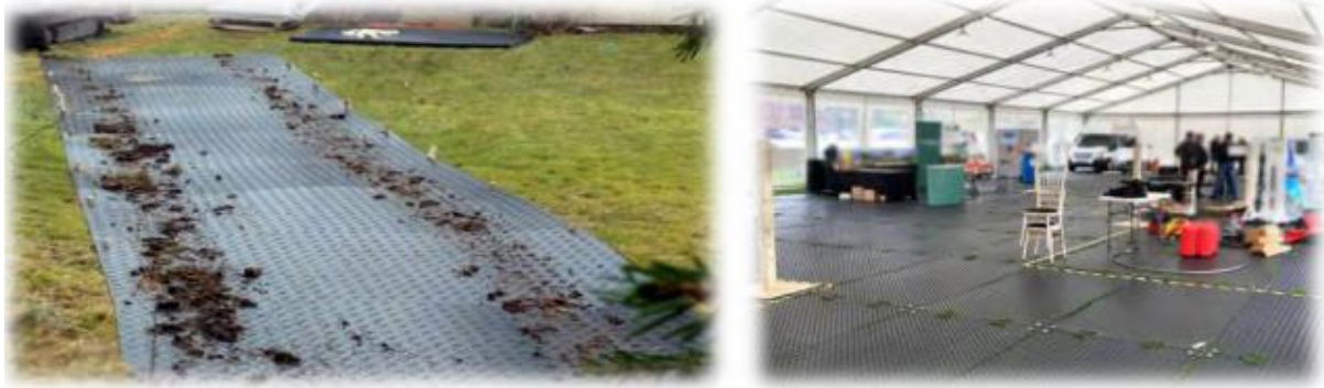
Figure 4: example of temporary ground protection boards to protect against footfall and light plant. (Multi Matts, n.d.)
