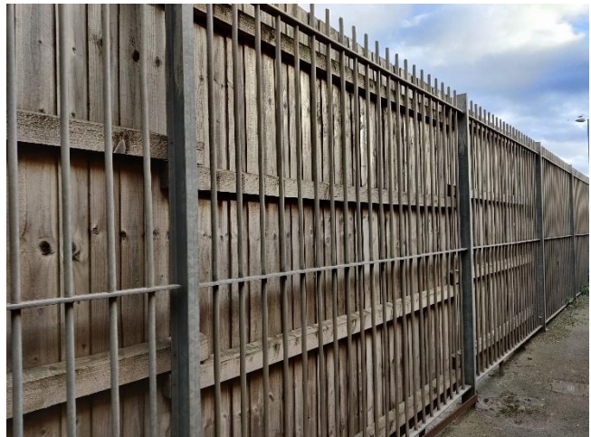
Photo 4: Metal and timber panel fence at the west site boundary.
