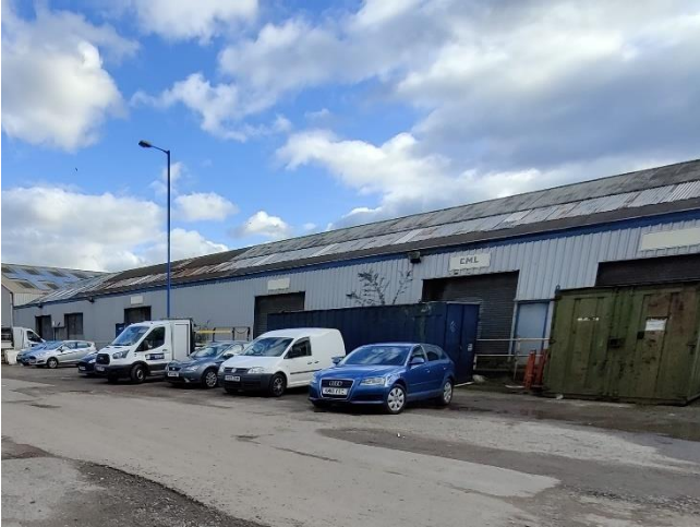
Photo 5: North elevation of B1.
