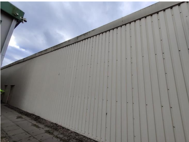
Photo 9: East elevation of B2.
