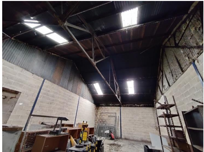
Photo 8: Typical internal view of B1.
