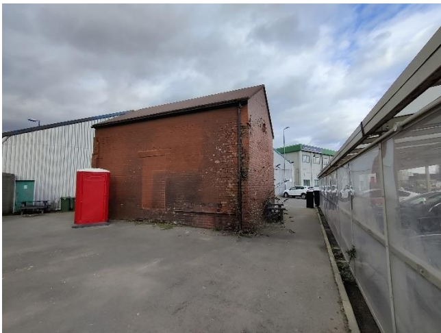
Photo 15: South and west elevations of B3.
