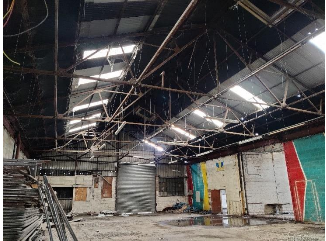
Photo 12: Typical internal view of B2.
