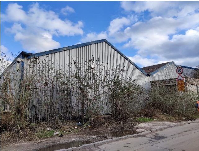
Photo 7: West elevation of B1.
