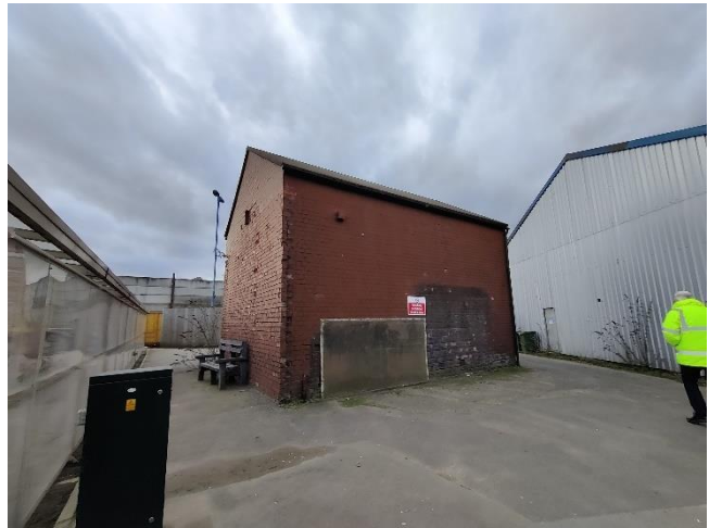
Photo 14: East and south elevations of B3.
