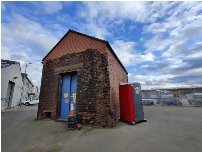
Photo 13: North elevation of B3.
