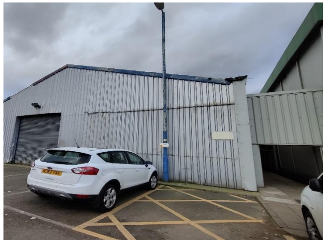
Photo 10: South elevation of B2.
