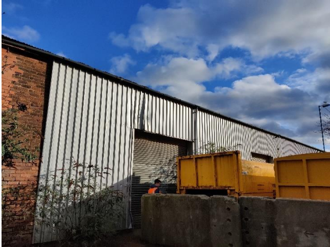
Photo 11: West elevation of B2.
