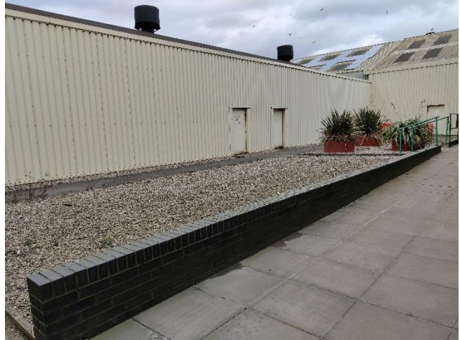
Photo 6: South elevation of B1.
