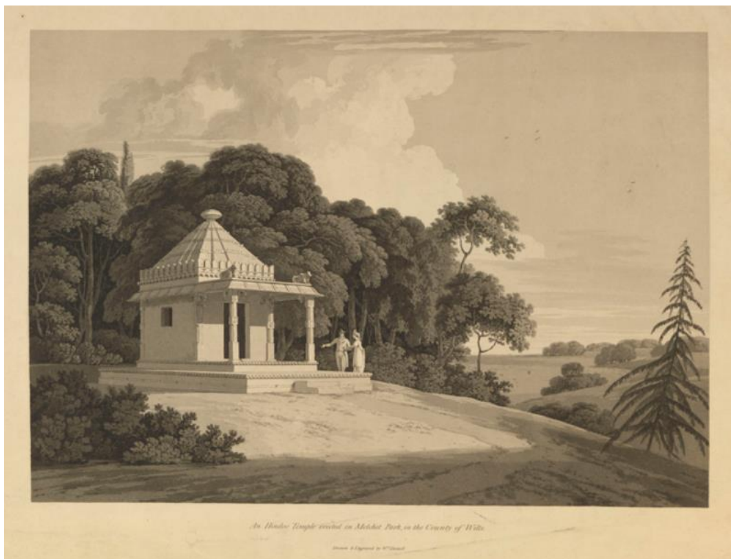
Figure 4: Sketch, by William Daniell, of the temple in Melchet Park © Royal Collection Trust
