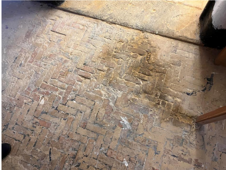
Figure 23: Brick herringbone flooring present within the former Stable Block/Coach House
