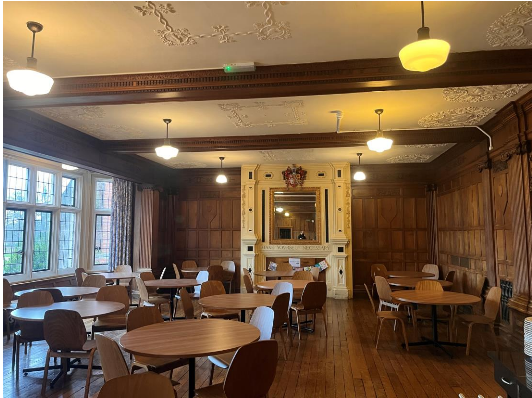
Figure 20: View within the dining room with wall panelling, timber floors and enriched moulded ceiling
