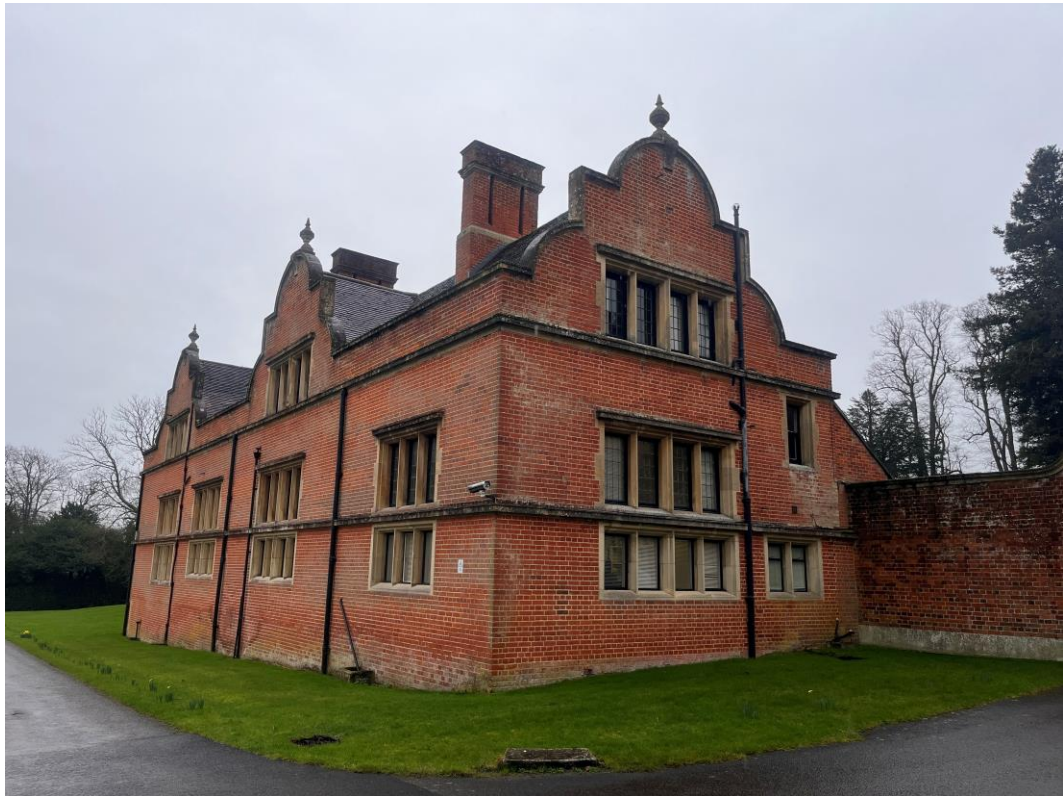
Figure 2: The former Stable Block/Coach House at Melchet Court, St Edward's School
