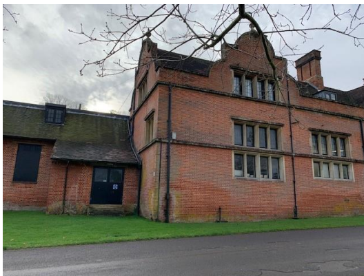
Figures 13 and 14: Single storey element of the former Stable Block/Coach House as seen from the north (left) and south (right) with modern brick infill
