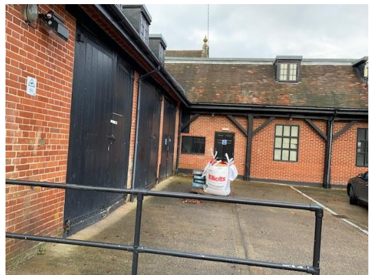
Figures 13 and 14: Single storey element of the former Stable Block/Coach House as seen from the north (left) and south (right) with modern brick infill
