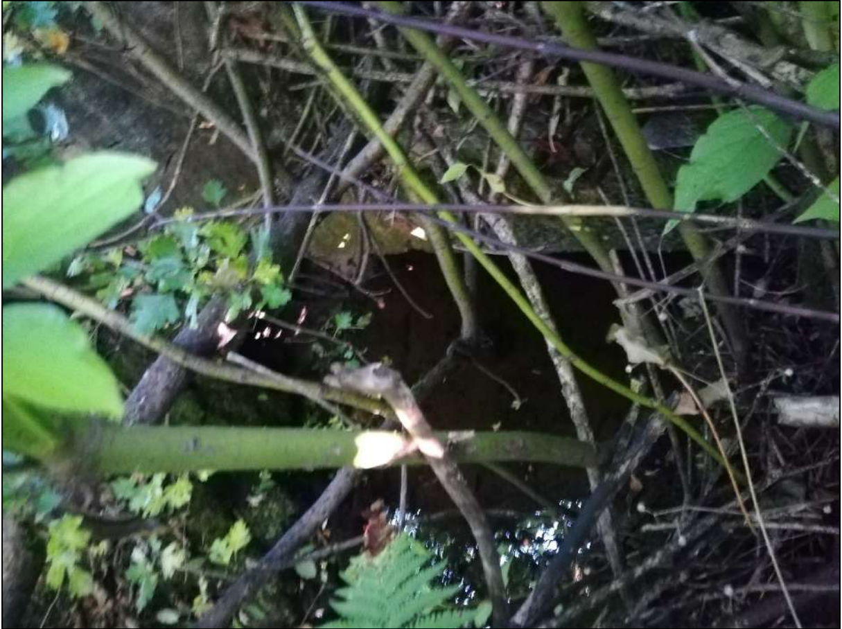
Photo 7: Outlet 1 just downstream of Beith Rd
