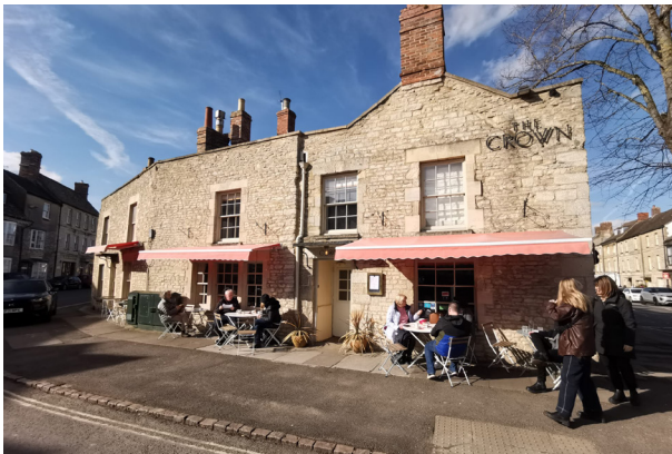
Fig. 2.1 View of awnings fixed to High St elevation.
