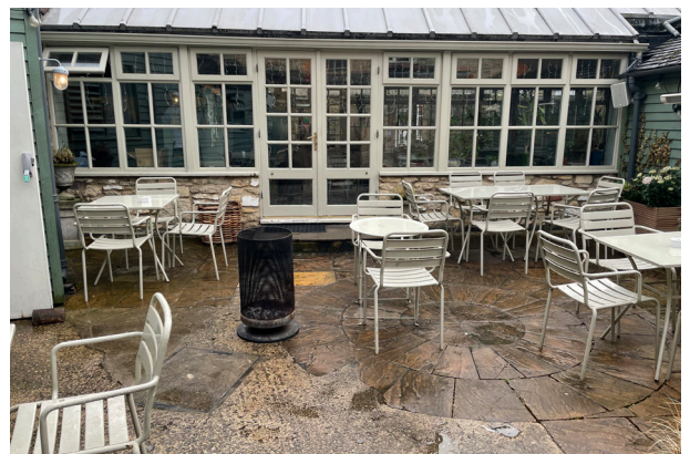
Fig. 2.6 View of coarsed rubble limestone wall and timber painted windows to Courtyard.
