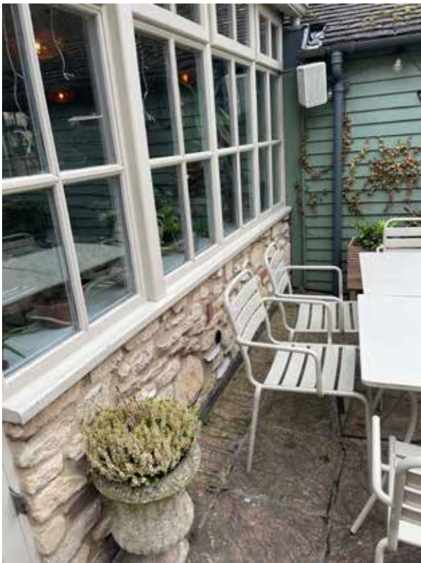
Fig.2.5 View of coarsed rouble limestone wall and timber painted windows to Courtyard.
