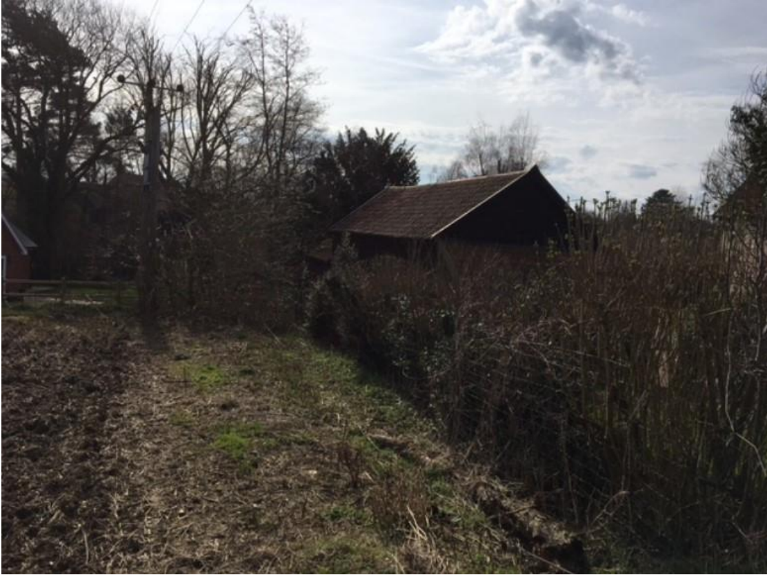
Rear Elevation, from field looking South West
