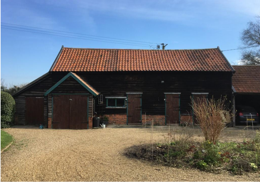
Front Elevation of Outbuilding (West)
