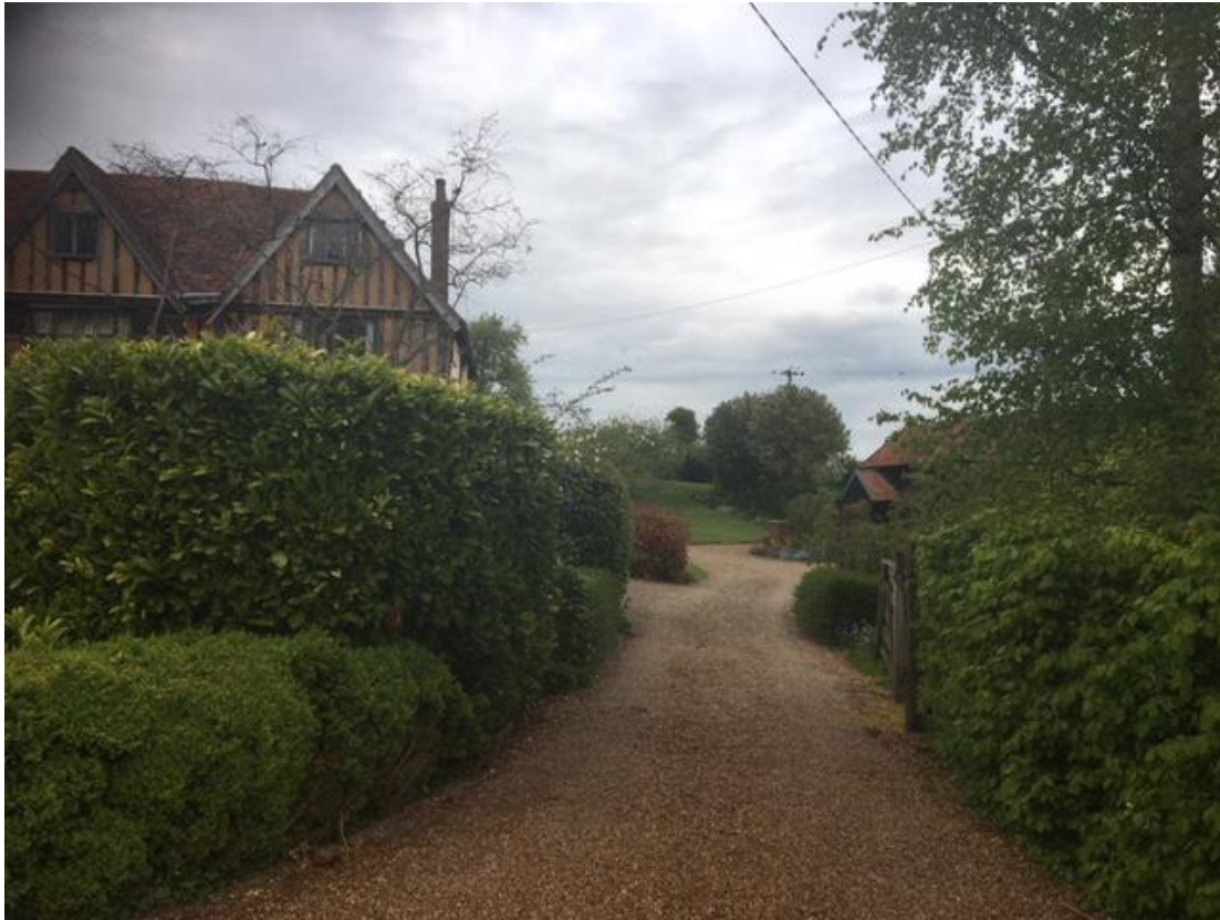
Outbuilding from east drive access, looking North
