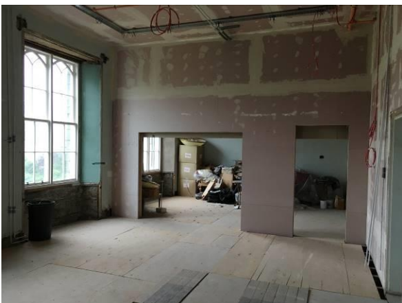
Second floor – South apartments, looking west
