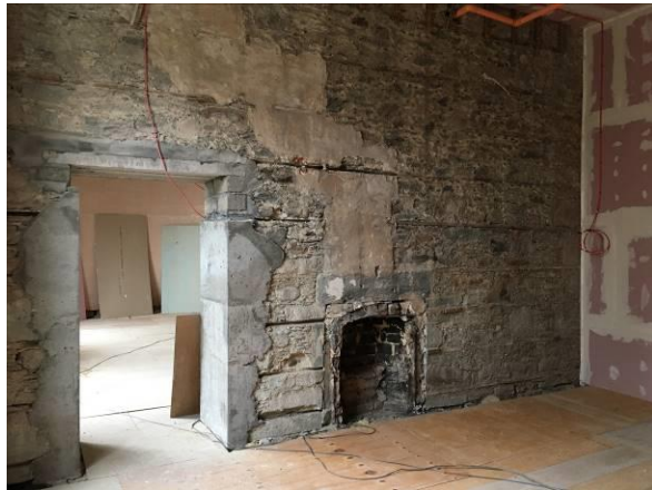
Second floor – Fireplace and existing masonry wall
