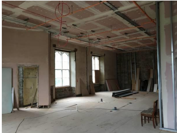
Second floor – North-West apartments, looking east
