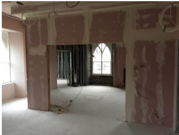
Third floor - South -West apartment, looking west
