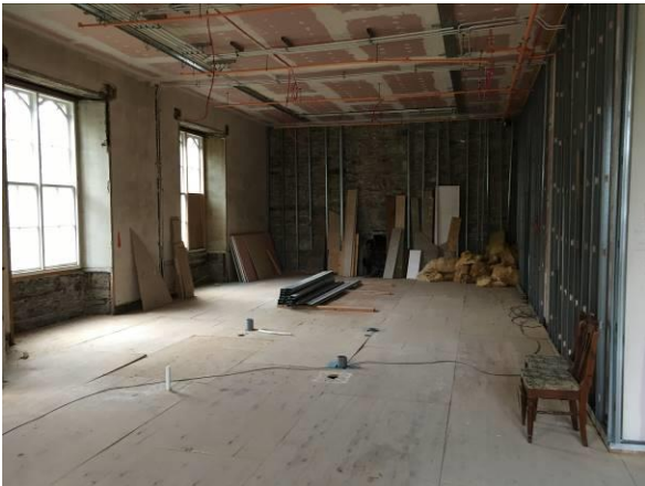
Second floor – North-West apartments, looking east
