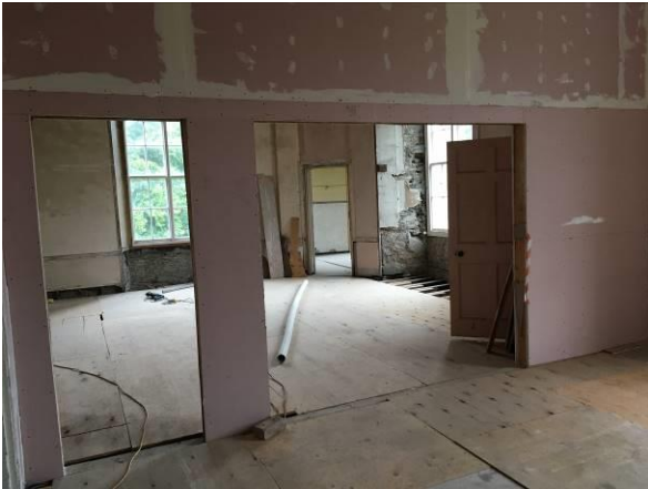
Second floor – North-East apartments, looking north
