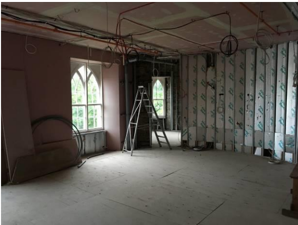
Third floor - North-West apartment, looking north
