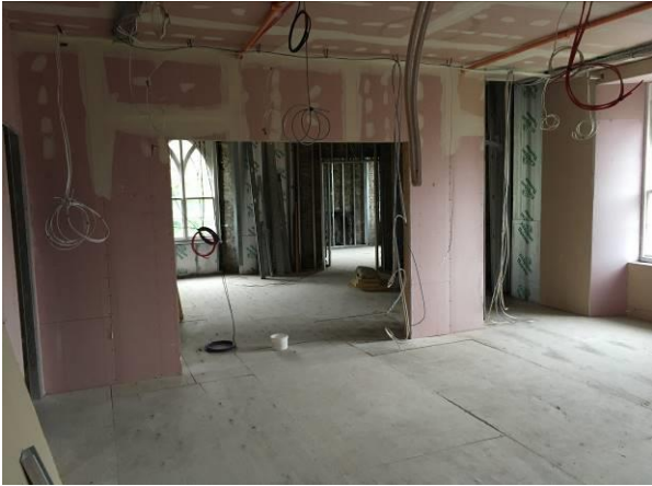
Third floor – North-East apartments, looking north
