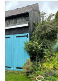
Barn as existing with hinged and sliding doors
