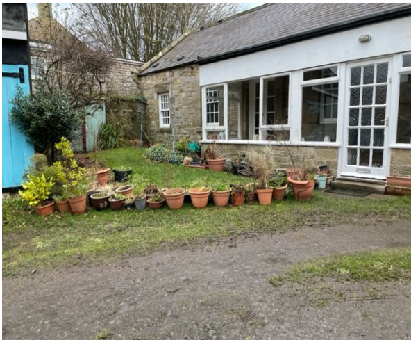
View of tracks adjacent to barn and sun room
