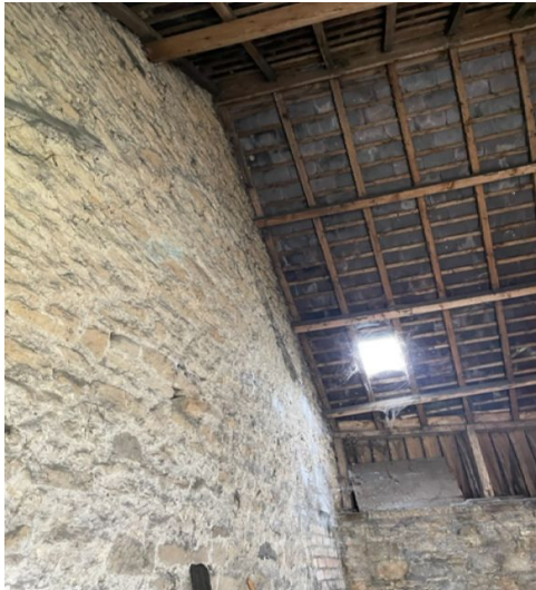
Existing barn interior
