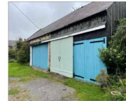
Barn as existing with hinged and sliding doors
