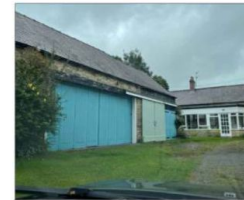
Barn as existing with hinged and sliding doors
