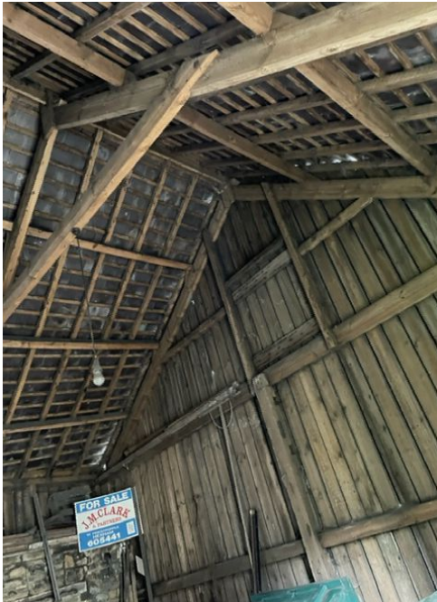
Interior of existing barn
