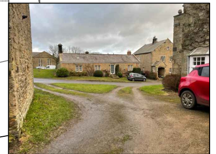
View of access track and car in parking space 1 for Kirsopp House
