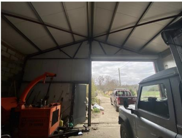
Picture 15: Inside section A (B1), facing west.
