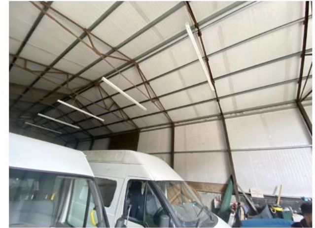
Picture 20: Inside section B (B1), facing northwest.
