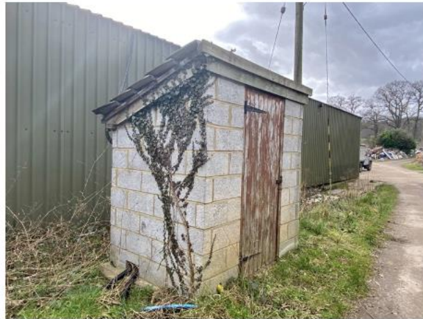
Picture 8: B2's northern and eastern elevations.
