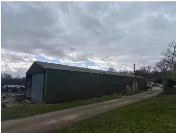
Picture 4: B1's northern and eastern elevations, as well as surrounding habitats.
