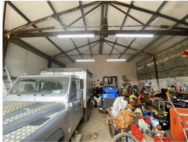
Picture 13: Inside section A (B1), facing east.
