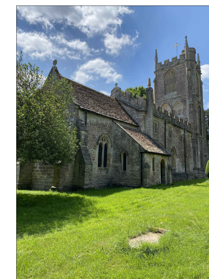
Church from north east
