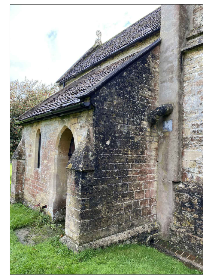
Existing asbestos flue and rendered blockwork chimney
