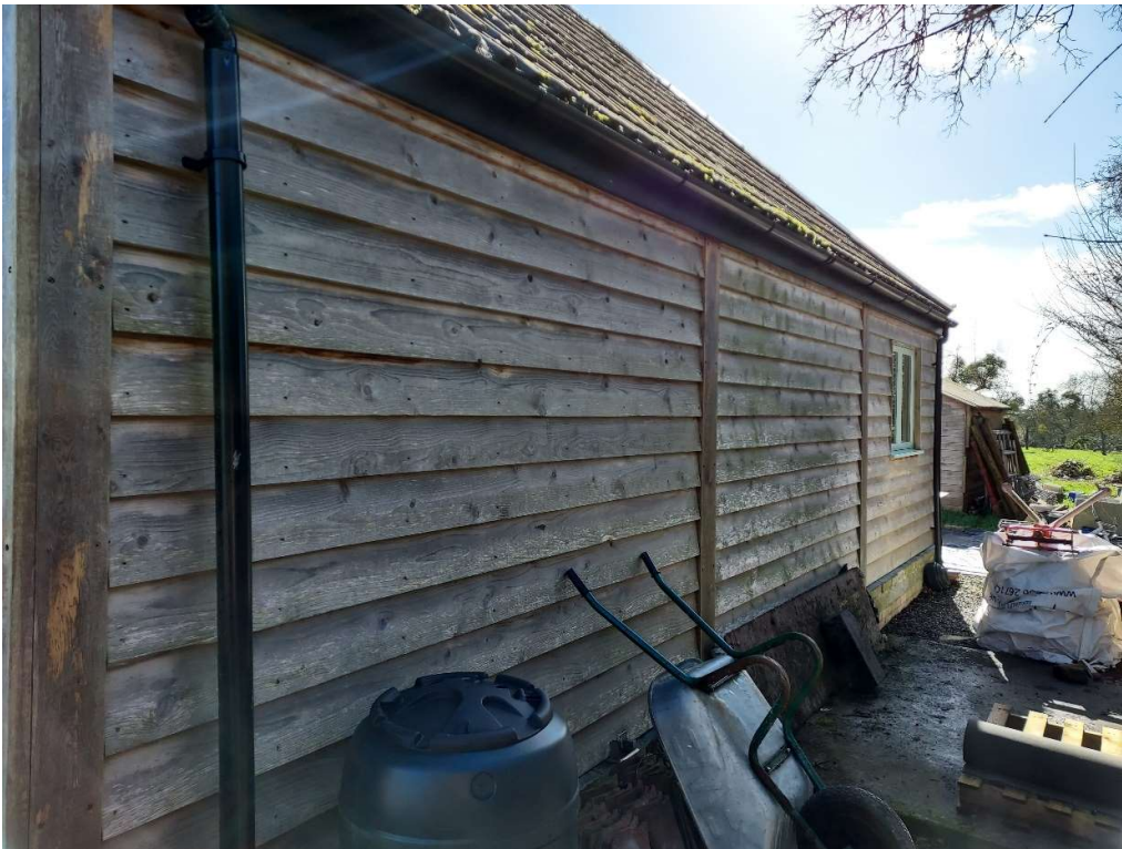
Image of the rear West elevation
