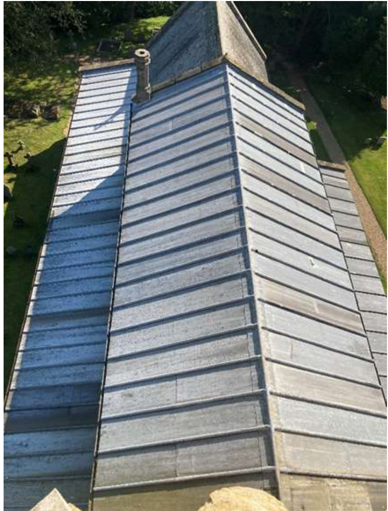
Figure 3: View of the church roof from the tower.
