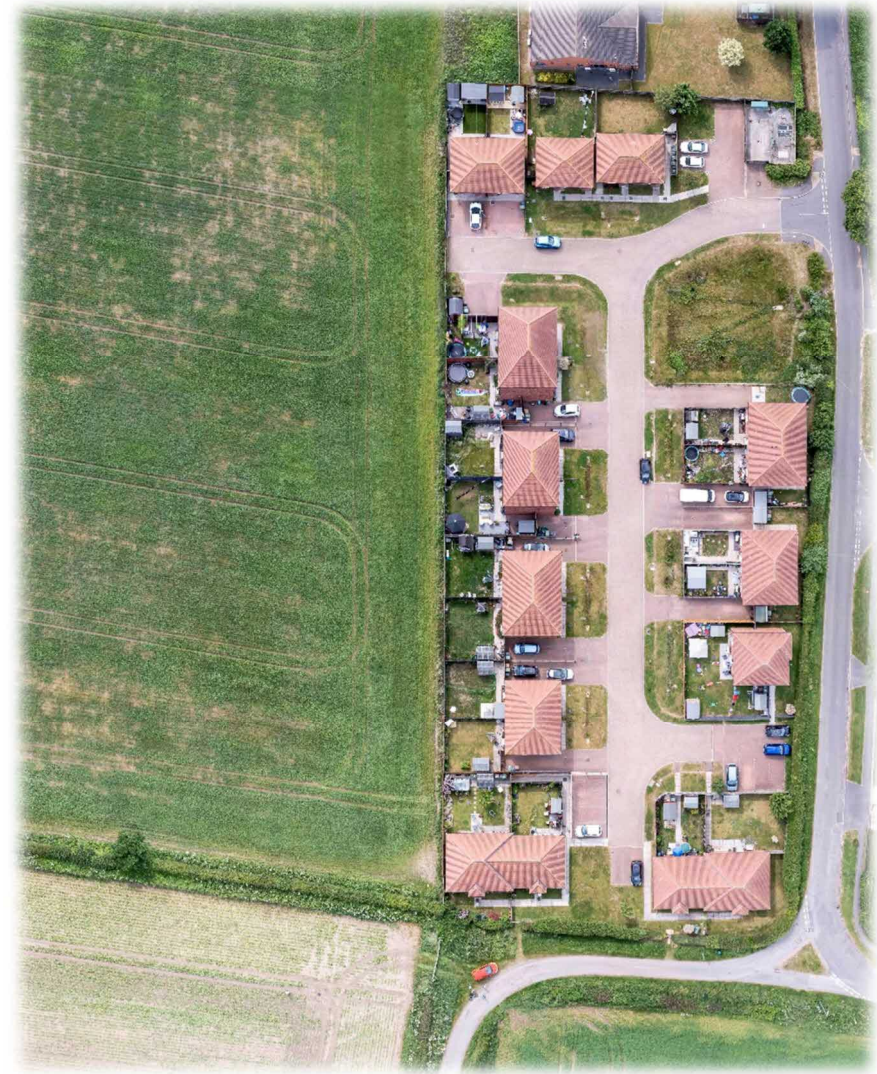
Aerial view of Vasey Close (right) and the application site (left)
