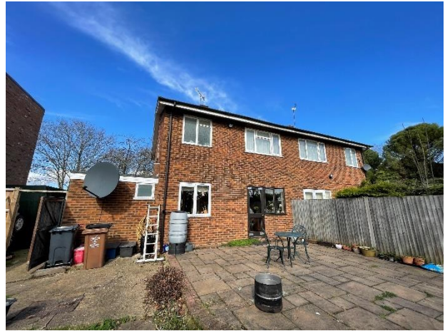
Photograph 2. 10a Burwell Road viewed from the south-east.
