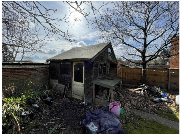
Photograph 4. The shed within the garden of 10a Burwell Road.
