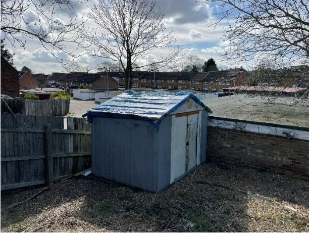
Photograph 7. The shed within the garden of 10b Burwell Road.
