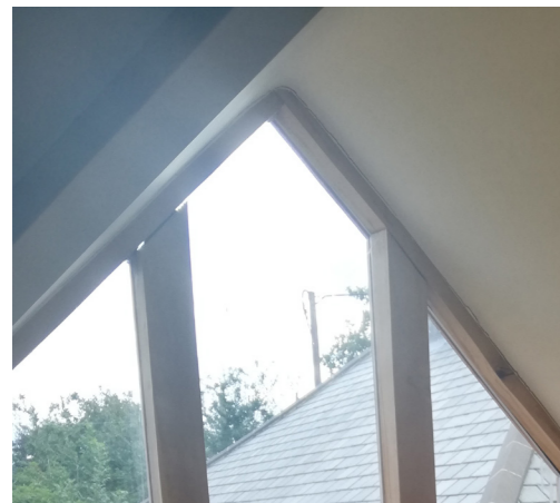
Interior view of the glazed gable construction quality
