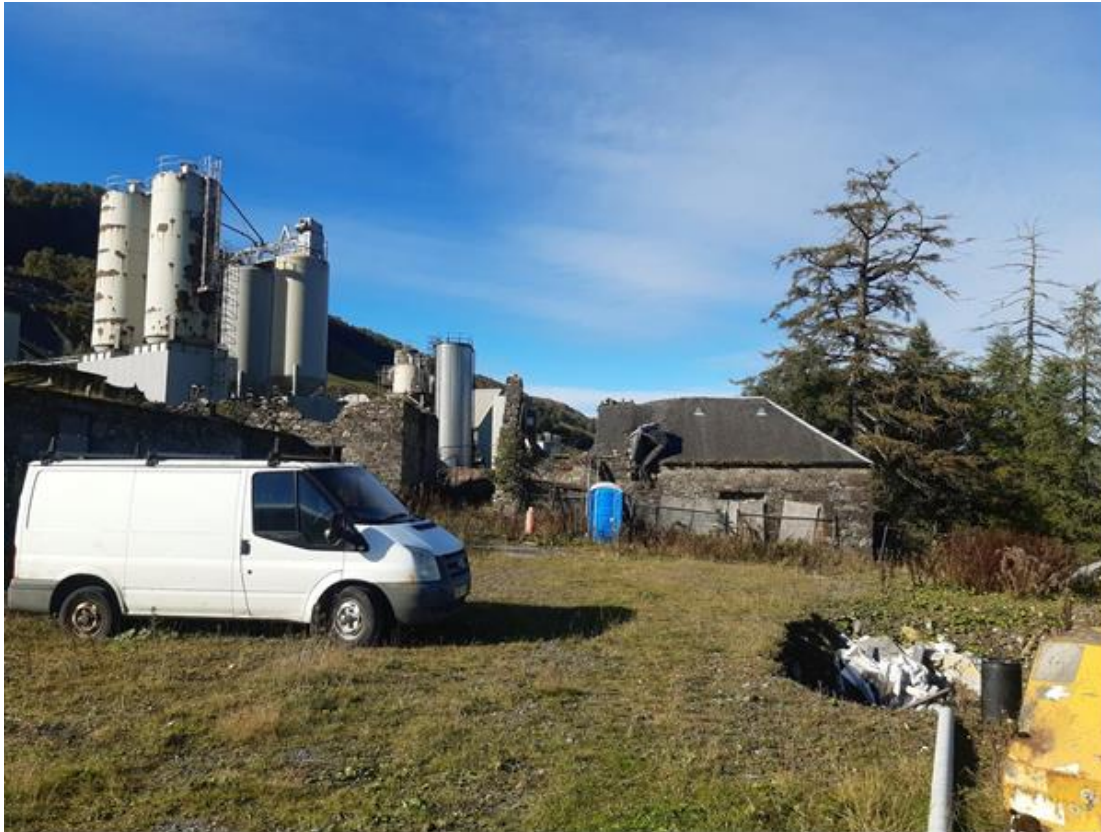
Plate 1 – View of Joiners Yard and existing Sheirglas Steading, looking west.
