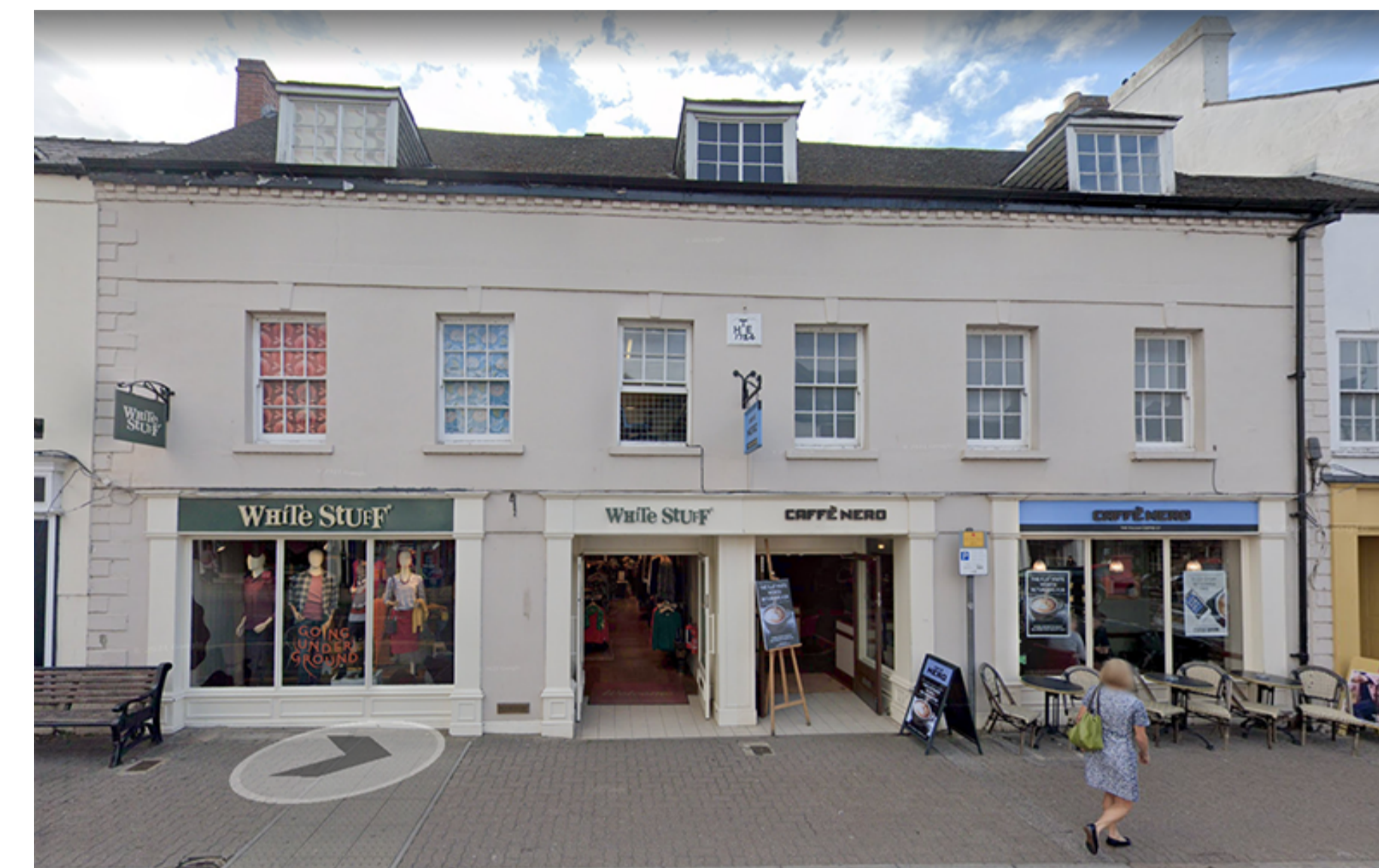
EXISTING SHOPFRONT PHOTO NTS
